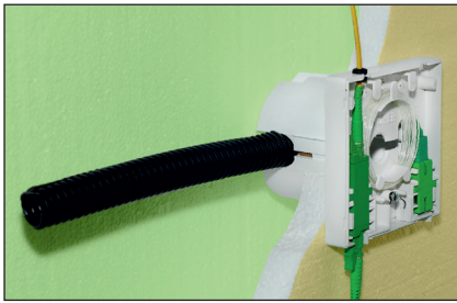
Installation of wall-mounted fibre optic outlet NGO-12
