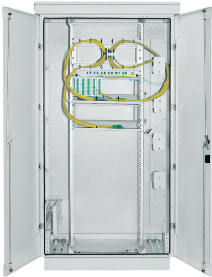
Street Cabinet PU-10 with FTTX equipment
