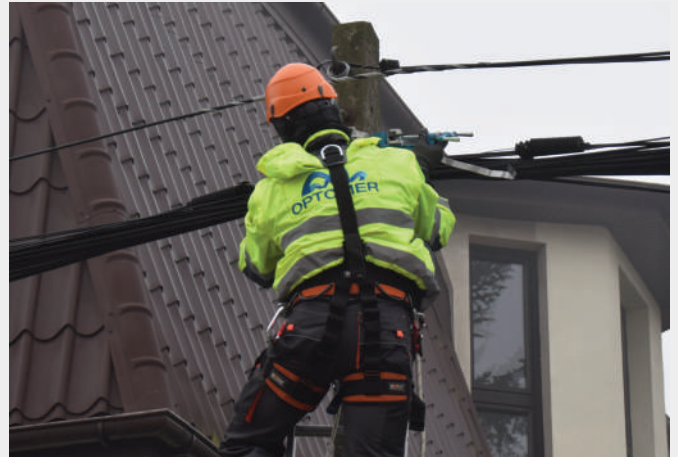
Example aerial network OPTOMER SKY SYSTEM + was built on the housing estate in Warsaw
