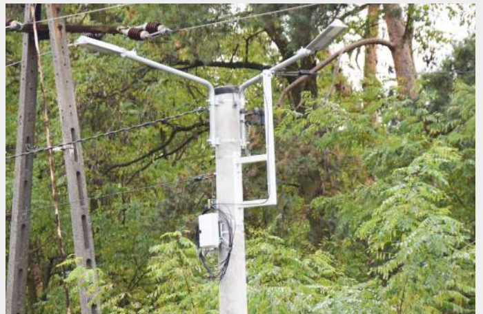
Bracket distancing cable from the pole.
