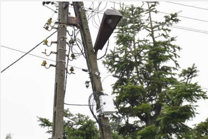
One of the main elements are MUF-8 optical closures with OSS-SZD-60 spare length frames.
