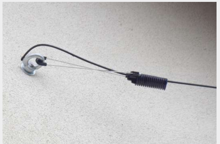
FTTH home drop with FSS-UO Anchor Clamp.
