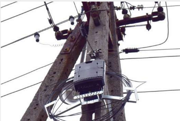
OSS_MUF-7 closures with OSS-SZD-80 spare length frames.
