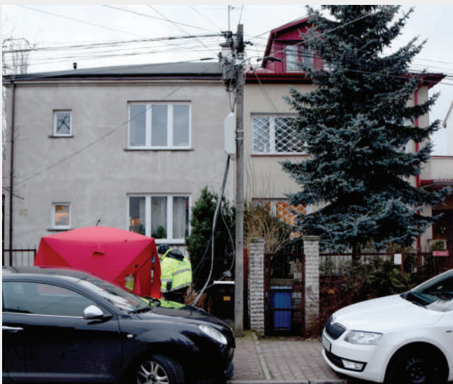
Fibre splicing in OSS+PSHN in a service tent.
