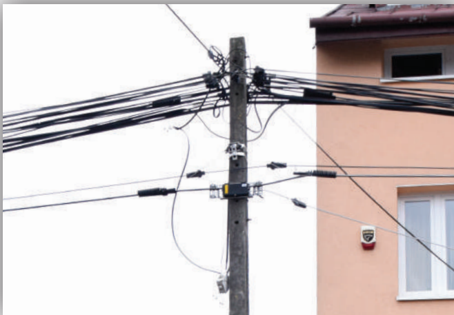
Using an aerial easy access cable OSS+KLD/ADSS enables quick and convenient customer connection.
