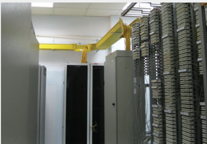
The central office equipment: central office cabinets, patchpanels, patchcords, adapters and cable ducts.
