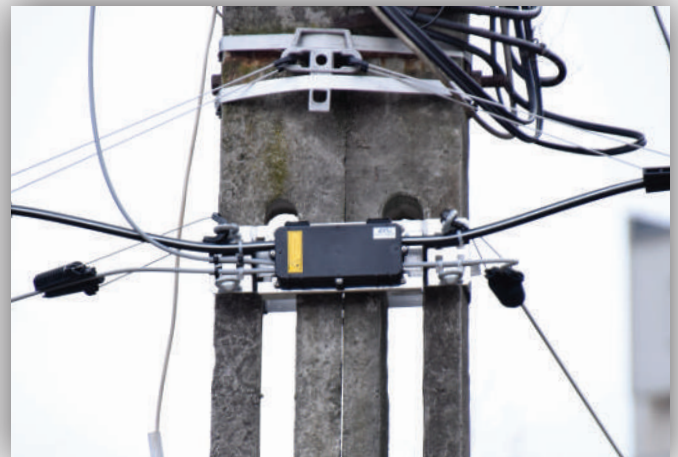
OSS+SD-KLD distribution box protects fibre module access point. The customer is connected with ADSS OSS+RA subscriber tube, by pushing or pulling the fibre.
