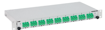
Nine FWDM multiplexers in 19 inch patch panel
